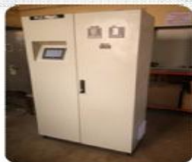
PLC Panel with 254 IO's
