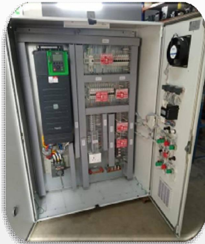
JAYATV-VFD WITH AUTOMATION PANEL
