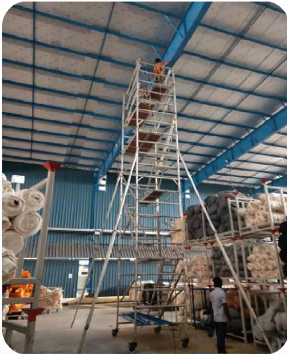
LED LITE & CABLE TRAY FIXING
