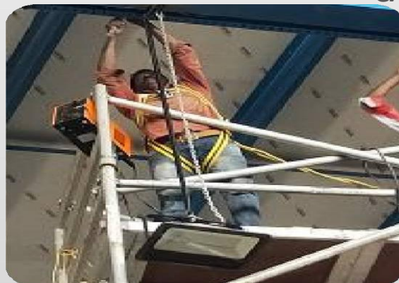
LED LIGHT FIXING
